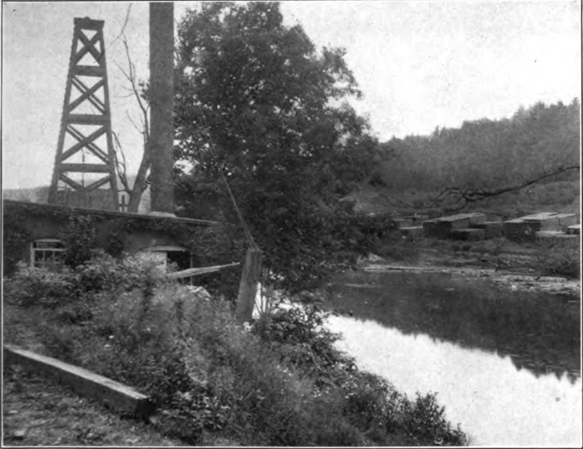
A. INTAKE OF PUBLIC SUPPLY AT BROOKVILLE, PA.
